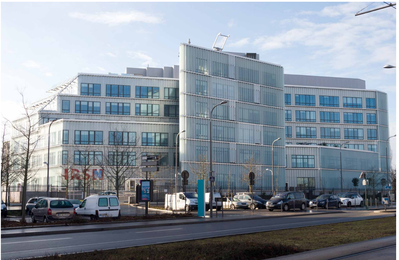
At Fontenay-aux-Roses, building 01 delivered in 2017 meets strict criteria for energy efficiency, functionality and comfort. It has "NF Tertiary Building" certification.
