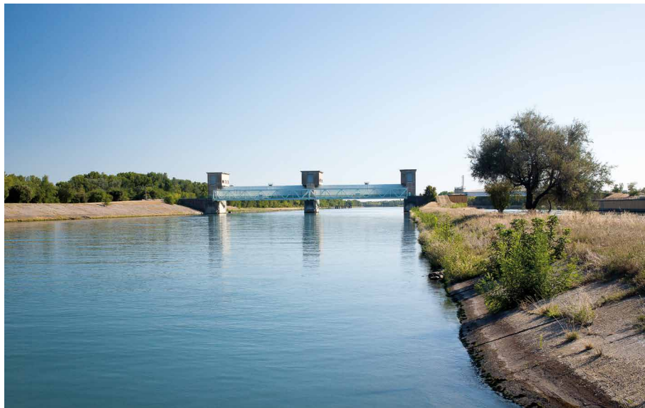
The dikes of the Donzère-Mondragon canal were reported by EDF and Orano (formerly Areva NC) due to a noncompliance with the safety baseline for the Tricastin site facilities.
