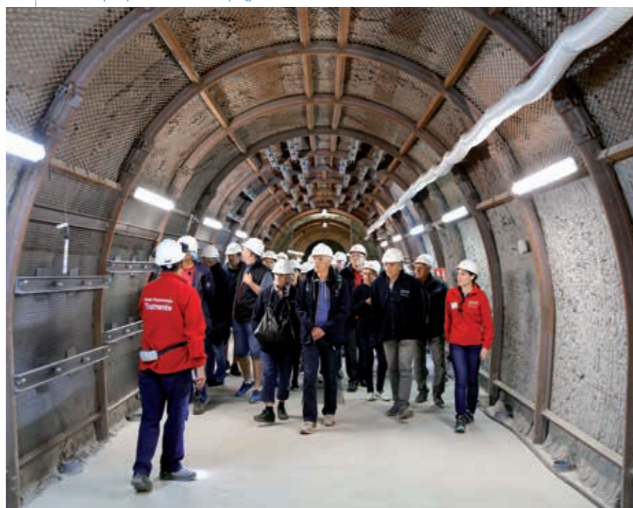
An IRSN expert presents research in progress in the West-2008 drift of the Tournemire tunnel.
