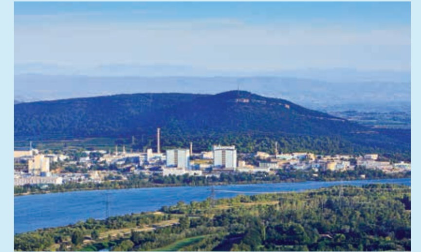
General view of the Marcoule site (Gard).
