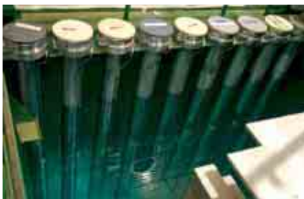
PHEBUS reactor: test device storage pit.
