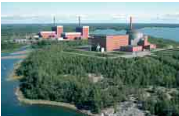
The EPR project in progress on the Olkiluoto site in Finland.
