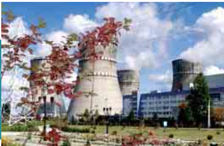
The Rovno plant in Ukraine.
