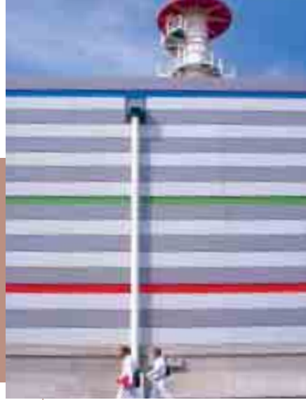
Melox MOX fuel manufacturing plant at Bagnols-sur-Cèze (Gard).
