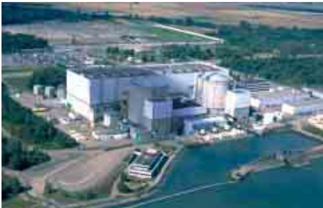
Aerial view of the Fessenheim nuclear power plant (Haut-Rhin).
