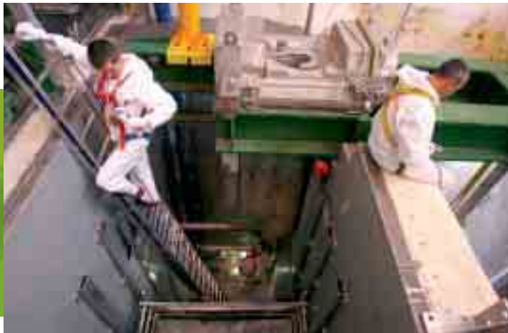
Storage tank for CABRI installation test devices.
