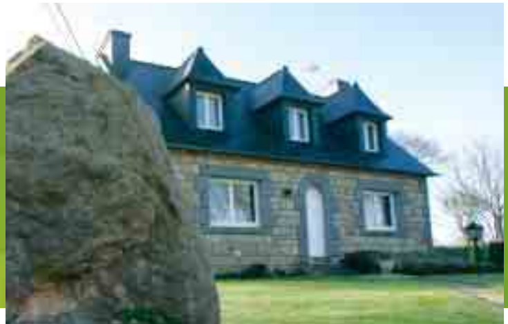
Granite house in Kersaint (Bretagne) where the Institute conducts experiments to further understanding of the circulation of radon in the home.
