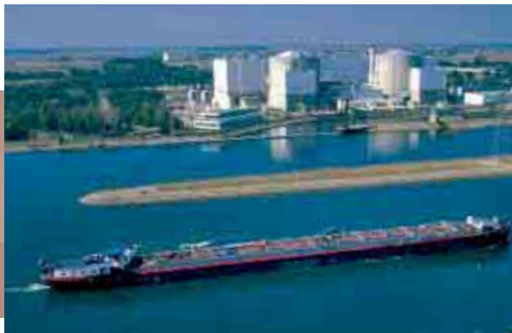
The Fessenheim nuclear power plant (Haut-Rhin).
