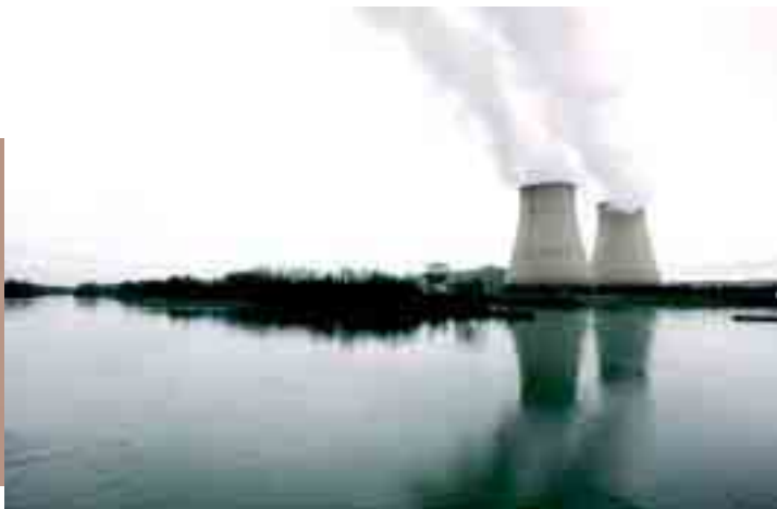
Power plant at Belleville-sur-Loire (Cher).
