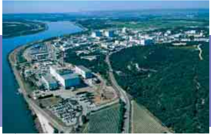
Aerial view of the Marcoule site (Gard).
