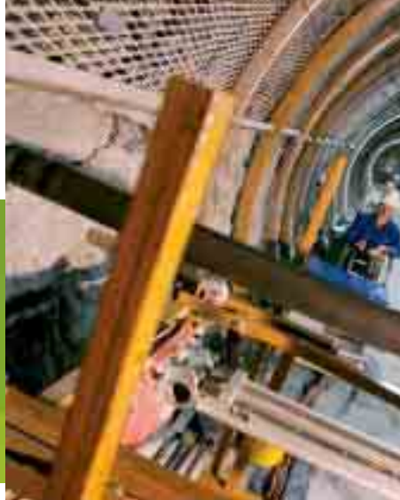
Dry boring in a gallery of an experimental tunnel at Tournemire (Aveyron).
