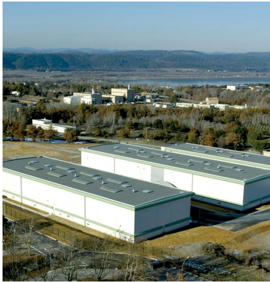
The CEA decided to install a new facility for processing and storing type B, low and medium radioactive waste. This new facility is the CEDRA project, "Radioactive waste conditioning and storage".
