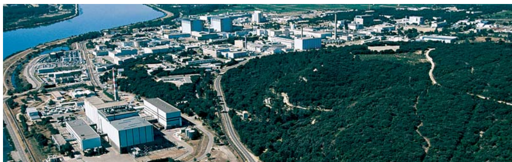
The Marcoule facility.
