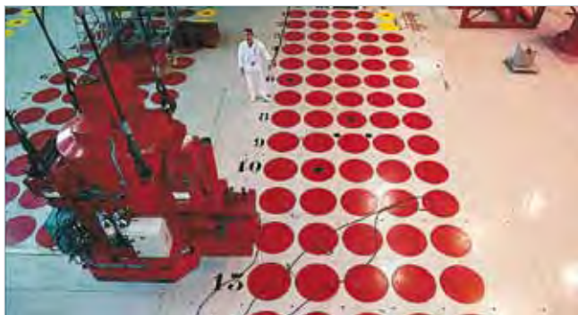
Interim vitrified waste storage. View from above the shafts (Marcoule).
