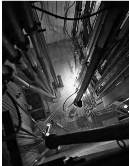
Figure 5.3. View of the SILOE reactor core. @ CEA.
