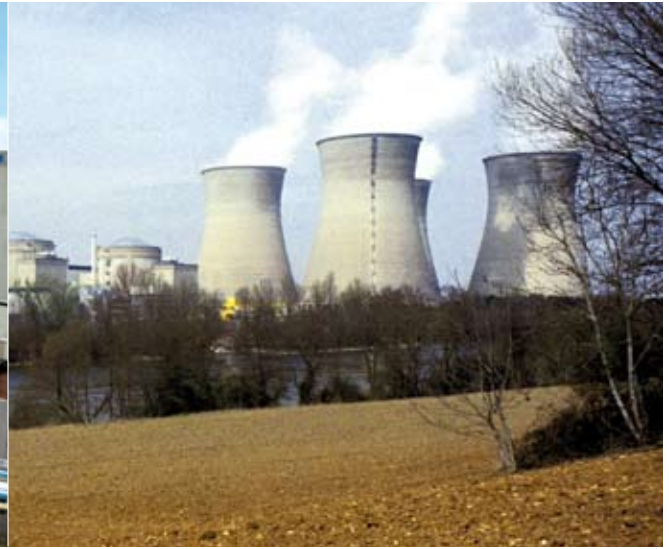
The Bugey site in eastern France.
