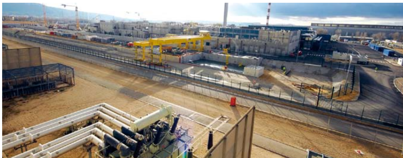
The Georges Besse II plant for uranium enrichment, using ultracentrifugation to produce nuclear fuel.
