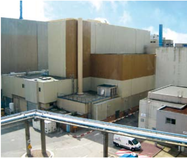
Dismantling the high-oxide-activity unit at the La Hague plant.
