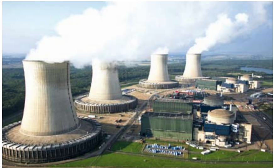
Cattenom nuclear power plant.
