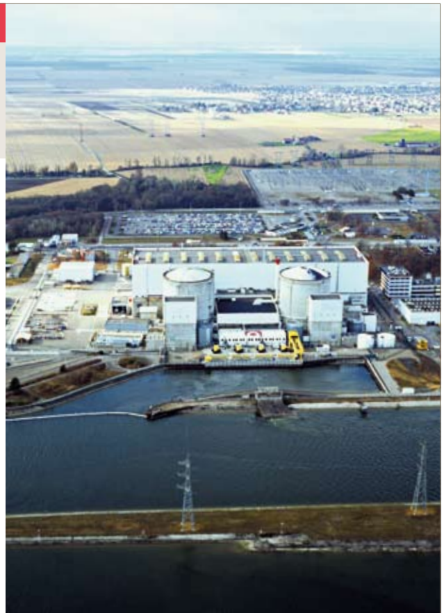
Fessenheim nuclear power plant.
