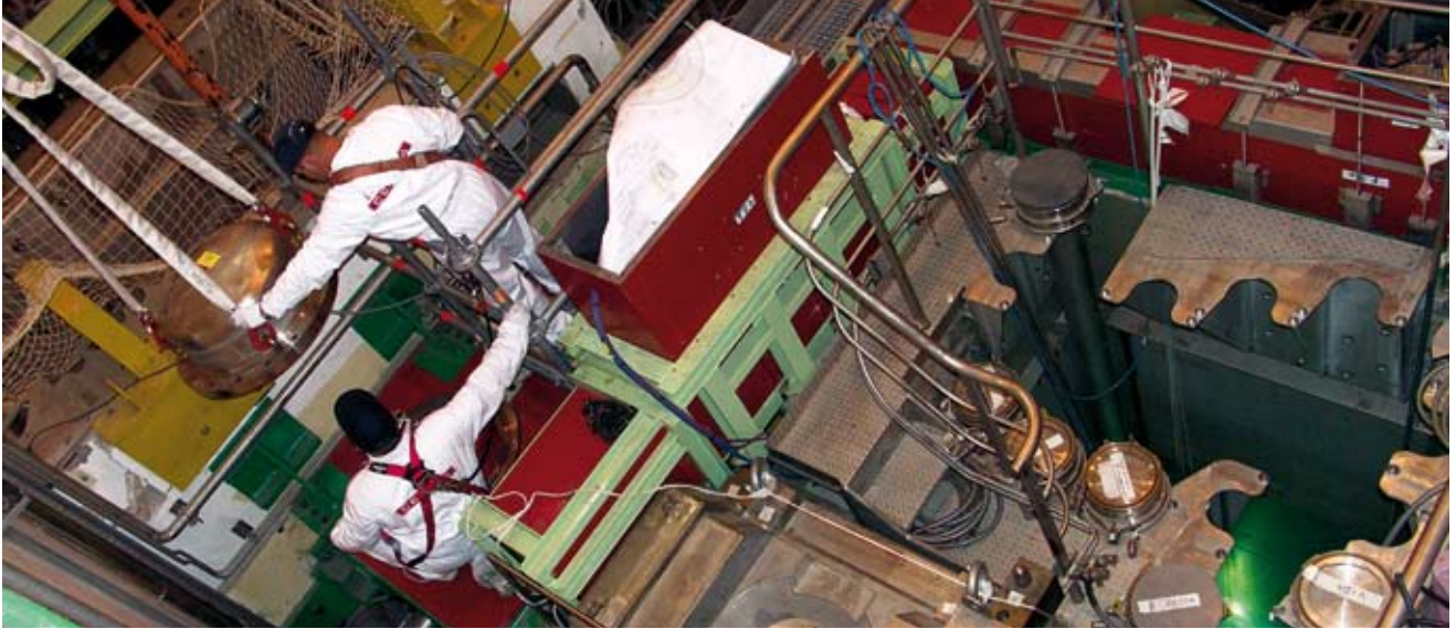
Renovating the CABRI experimental reactor.
