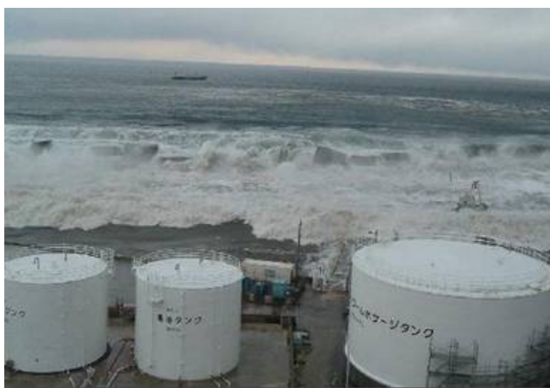
Figure 3-7 - Submersion de la digue de Fukushima Dai-chi (source TEPCO)
