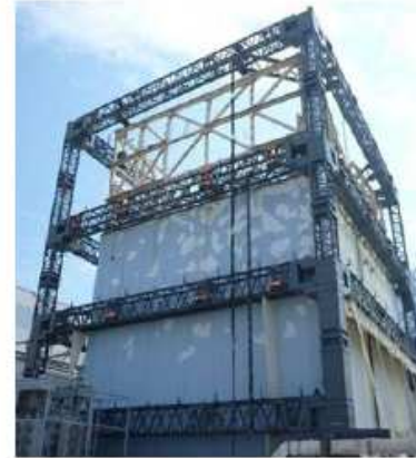
Completion of steel framing
