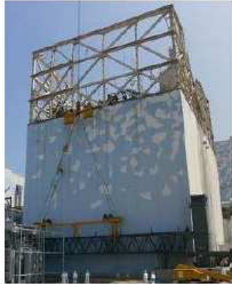
Start of steel framing
