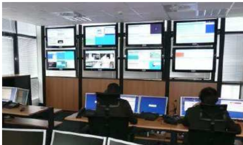
Figure 12 : Salle de supervision (Thalès - monitoring center)
